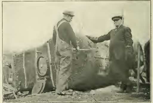
Boiler Being Cut with the Oxy-Acetylene Torch for Scrapping.
